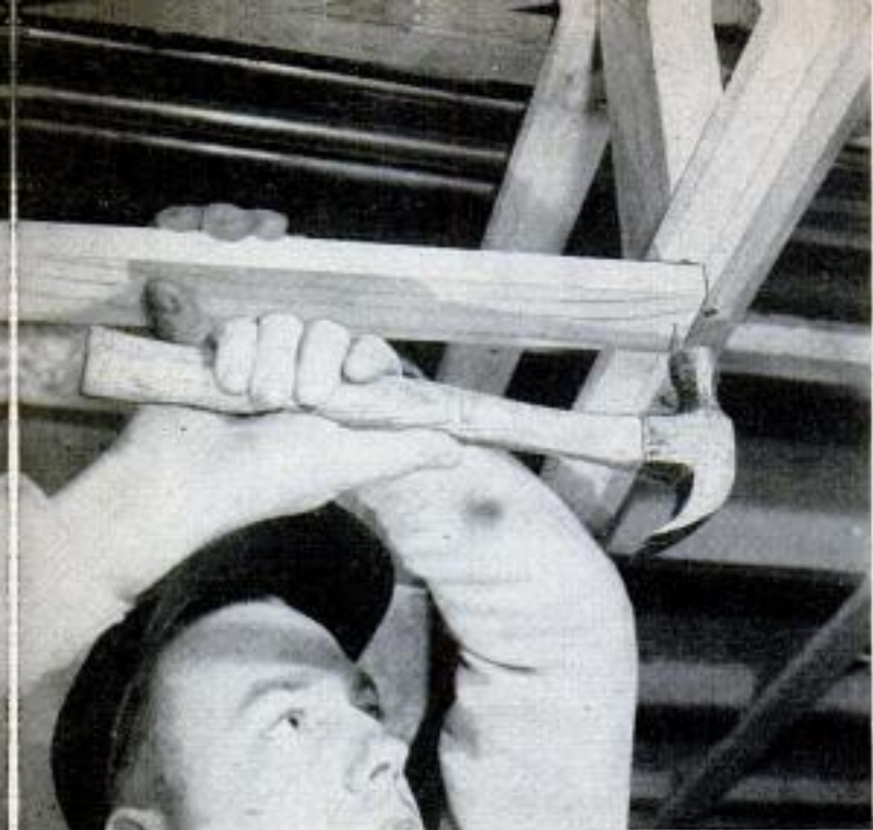
Boxing along both sides of room is used to conceal ducts and water pipes without lowering entire ceiling
